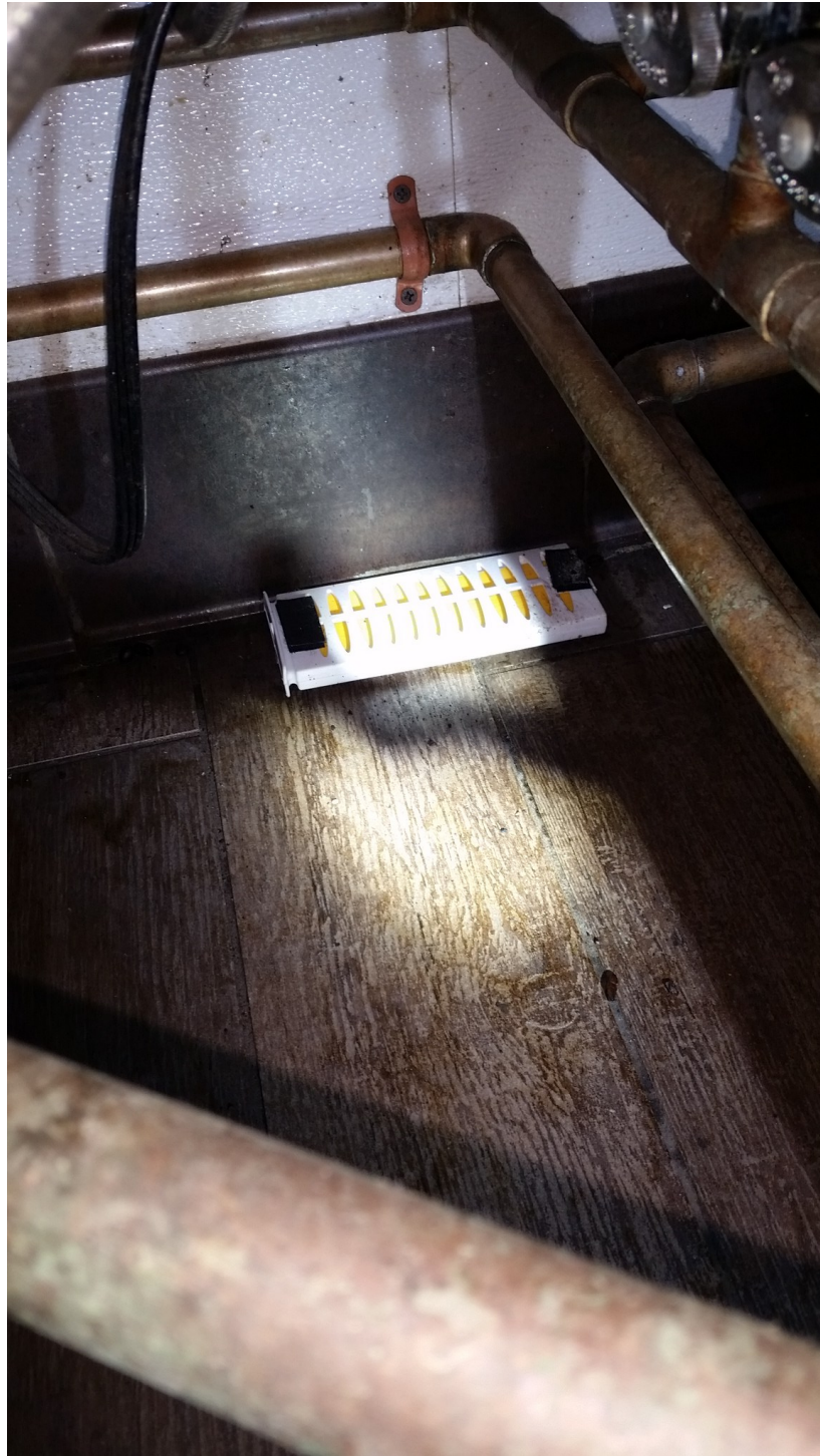
Manhattan Store (Mar. 8, 2016) DDVP No-Pest Strip Behind Sink Velcro Strips Used to Affix Out of Sight Are Also Visible
