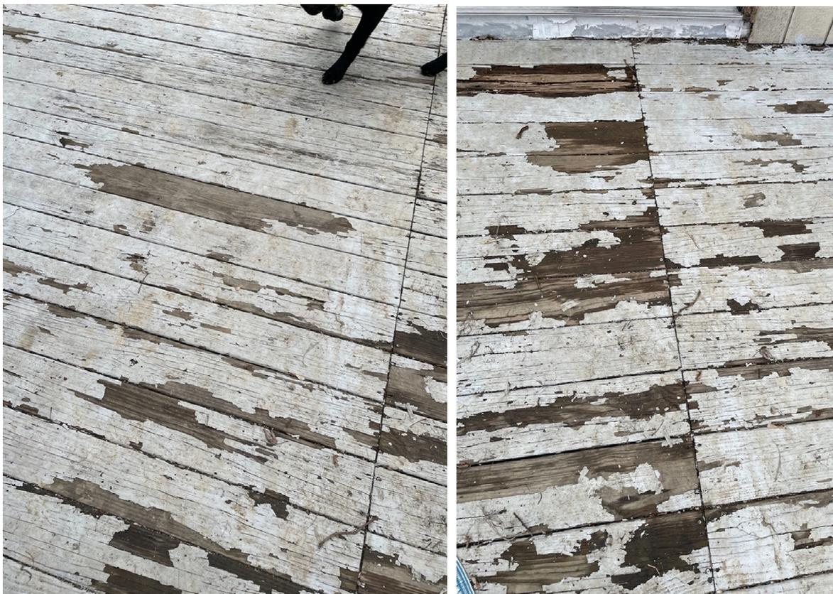
82. To date, Plaintiff's deck remains in a state of disrepair, as the Restore Products still crack, chip, strip, and otherwise fail and degrade.
